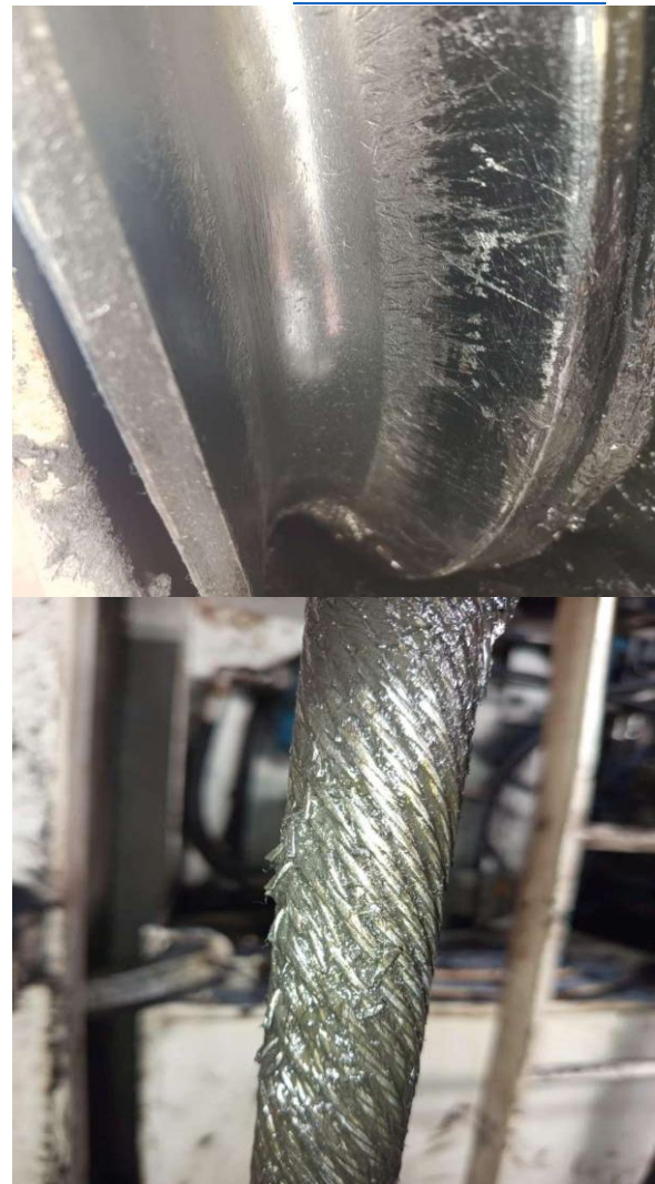
Figure 3. Imprint marks on sidewall of the sheave surface and failure mode of hoisting wire
