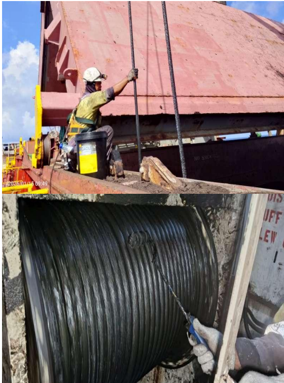
Figure 4. Manual application of lubrication the entire wire and the wire winding section on the drum
